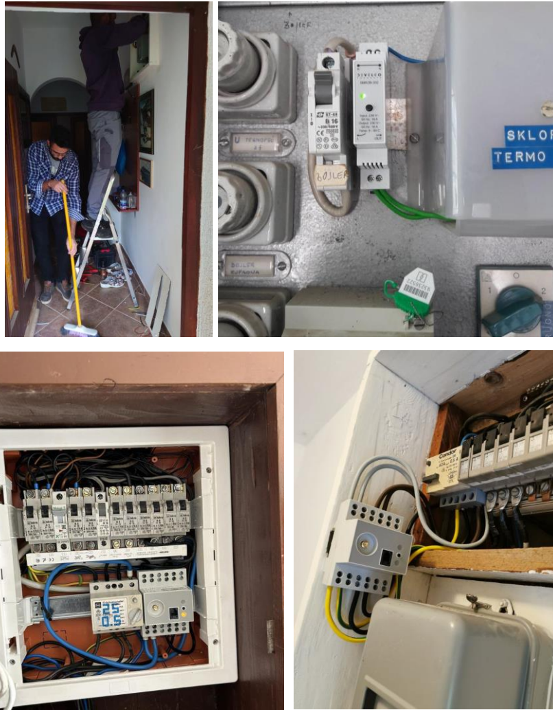
FIGURE 21: [CROATIA DEMO SITE] DWELLING INSTALLATION PROCEDURE AND INSTALLED SMART RELAYS AND SMART METERS
